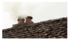
Check the top of the chimney - if you see smoke - adjust the air controls
